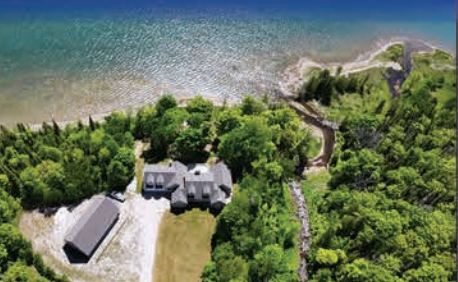
88 acres, private trout stream & 4,850 sq. ft. stone sided estate home MLS#2117008 - Manitowaning, $1,689,000
