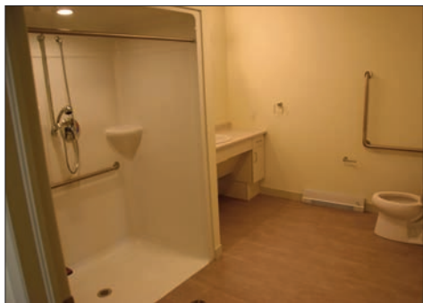
Two of the fully accessible units are equipped with larger doorways and accessible washroom and bathing facilities.
