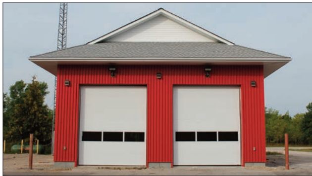
The new Billings fire hall is near completion.
