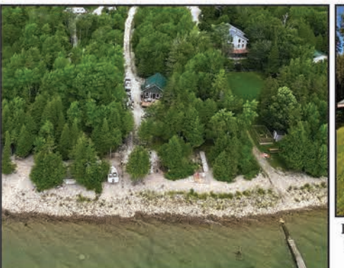
New-build under construction! Electrical service hooked up & ready for finishing to your liking! Seasonal cottage with an open kitchen/living area, walk-out to large deck! 3-bed & roughed in bath. MLS#2117839 - Manitowaning, $334,900
