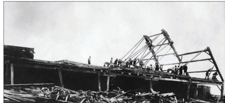
The first bent goes up! Photo of an undated barn raising near Thamesford, Ontario.
