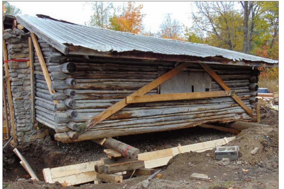
The Sheguiandah walleye hatchery building was built in approximately 1939.
