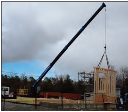
Construction started on the Billings township fire hall last week.
