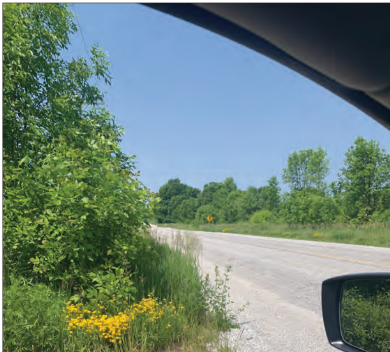
The roadsides along the Burpee Stretch have become heavily overgrown, providing a less than ideal sightline for vehicles driving down Highway 540.
