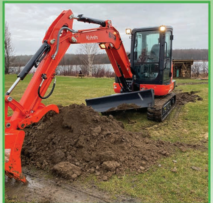
LOT CLEARING AND EXCAVATION
