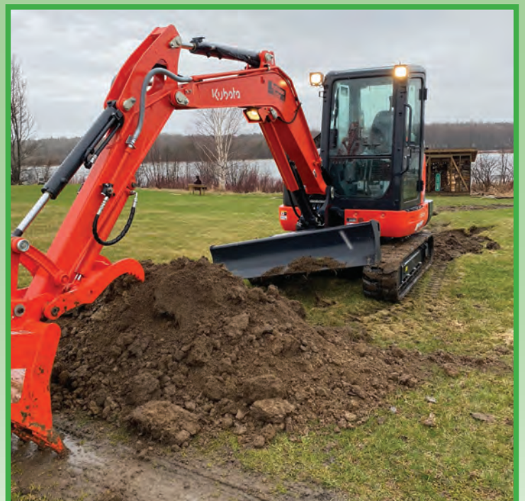
LOT CLEARING AND EXCAVATION
