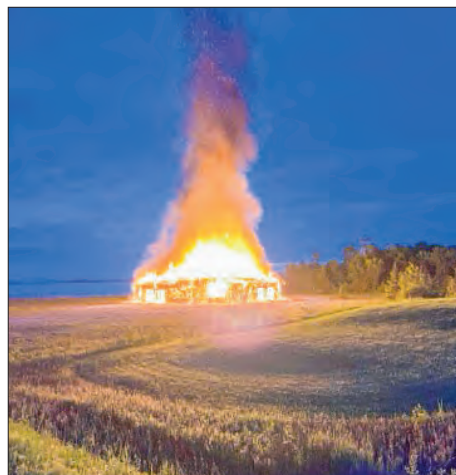
The Sheguiandah roundhouse fully engulfed, before fire crews arrived.
