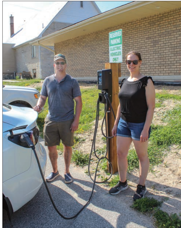
Brad and Anya Wright charge up their car at the electric vehicle station the couple paid for in Gore Bay. The unit was installed by the town.
