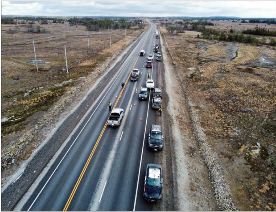
On November 24, members of the Manitoulin detachment of the Ontario Provincial Police (OPP), North East Region OPP traffic incident management and enforcement team (SAVE) in conjunction with the Ministry of Transportation and conservation officers from the Ministry of Natural Resources and Forestry conducted a five-hour Reduce Impaired Driving Everywhere program on Highway 6.
