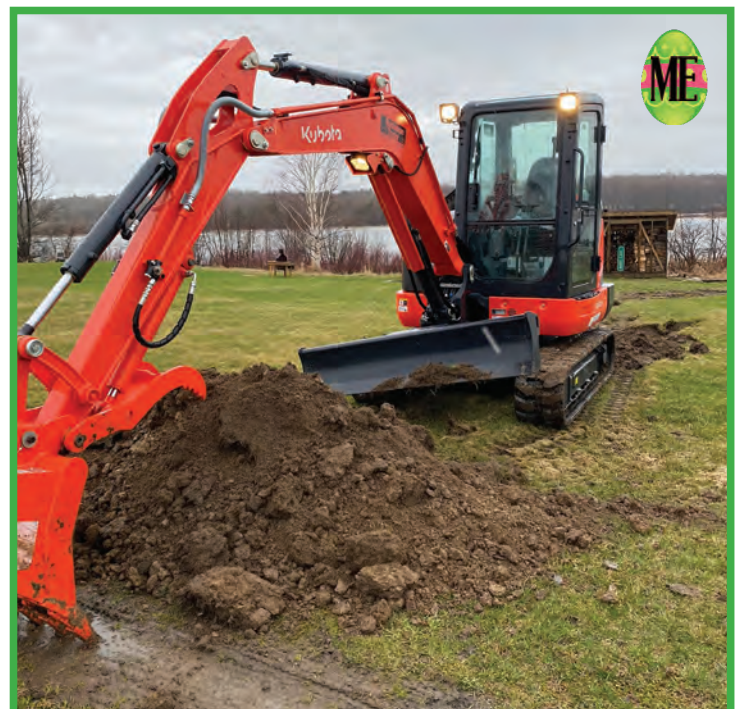
LOT CLEARING AND EXCAVATION
