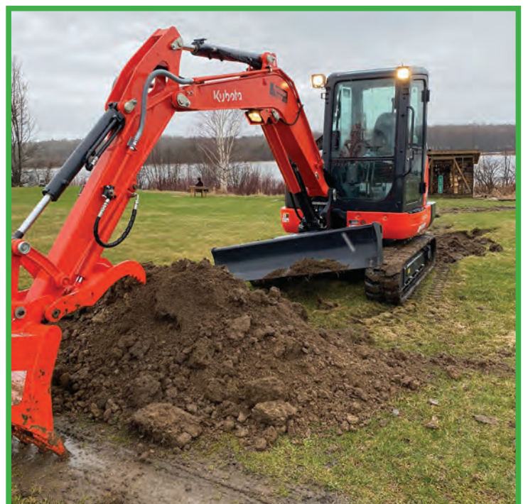
LOT CLEARING AND EXCAVATION
