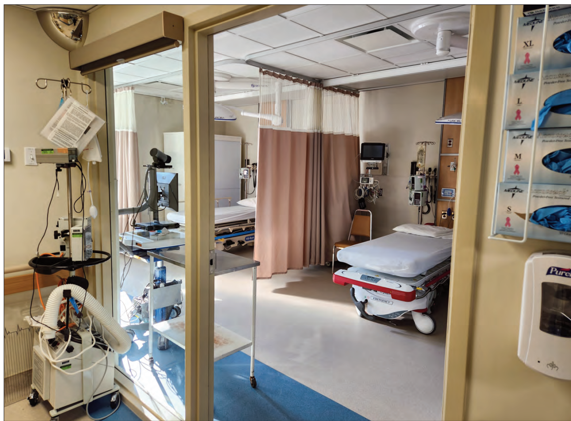
MINDEMOYA HOSPITAL HAS 'EMERGED' —the trauma room at the Mindemoya Hospital. Renovations and expansion of the emergency department at the hospital are now complete and the new site is in full use.
