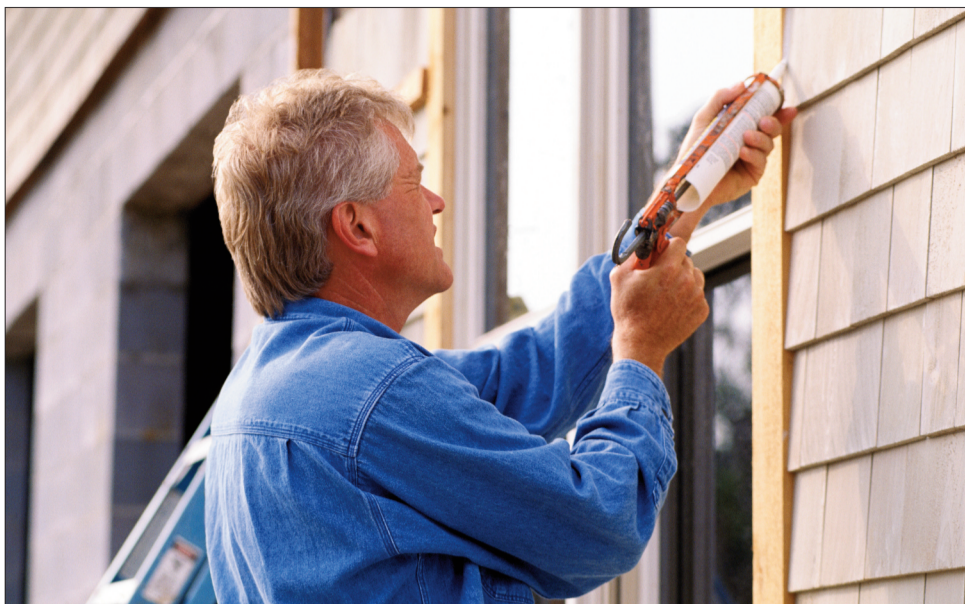
Caulking windows ensures a lack of home heat loss.
