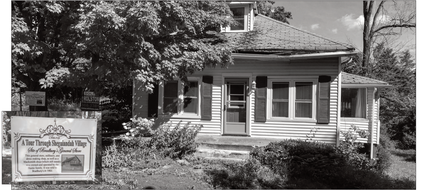
The Northeast Town will demolish a Robert Street home in Sheguiandah this fall to improve line-of-sight on a hairpin turn in the village. INSET: An historical marker notes its place on the village walking tour.
