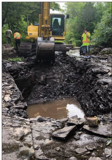
Part of the work in the Bass Lake Creek project involved digging a hole that was later covered by a thick layer of spawning gravel.
