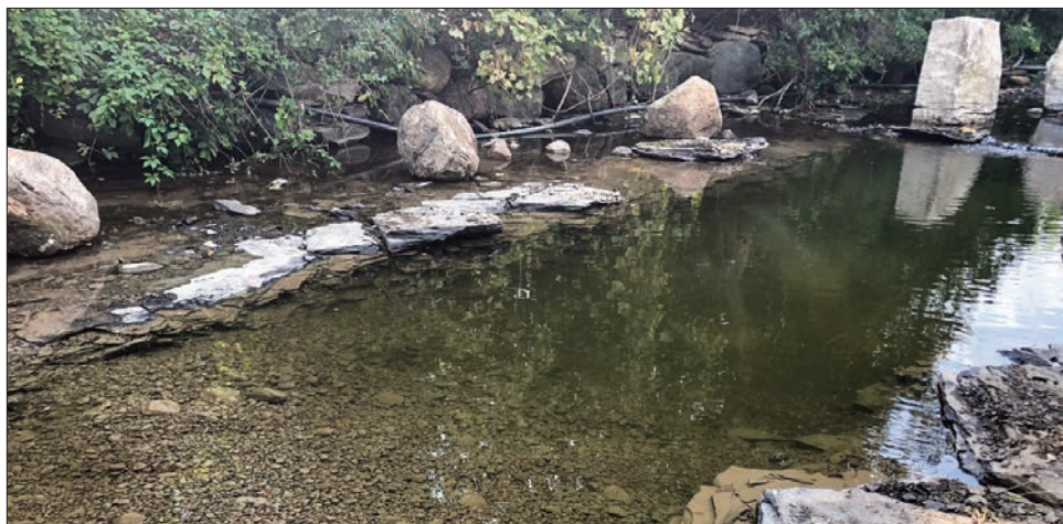
The finished pool adds depth to the creek and is lined with gravel that the fish can use when they swim upstream to spawn.
