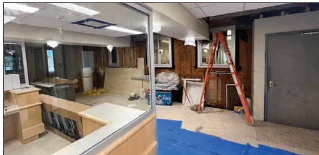
A peek at the emergency department renovations.
