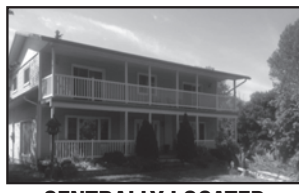
CENTRALLY LOCATED LITTLE CURRENT HOME
