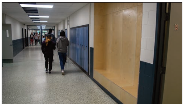
Some of the removed locker banks have been converted into wood-finished bench seating areas.
