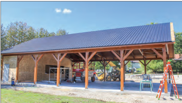
A new community pavilion is under construction in Gore Bay.
