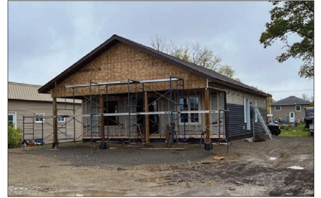
A new house is under construction on Vankoughnet Street.
