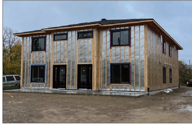
A four-plex on Vankoughnet Street is nearing completion.
