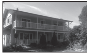
CENTRALLY LOCATED LITTLE CURRENT HOME
