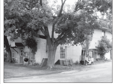
BLACKSMITH CENTRE on corner of Main & Meredith Streets w/4320 sq. ft. over 2 floors. Concrete building 36x60 ft. on fully serviced 39x127.6 ft. lot zoned core commercial. First floor garage plus business space & second level 4 & 1 bedroom apartments. $119,000 plus HST (1432)
