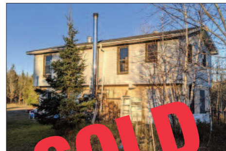
YONGE STREET COTTAGE on 7 ac. of forest near Government Rd. w/ private w/ year round access. Spacious raised bungalow 1400 sq. ft. w/640 of kitchen & dining at ground level & 760 on next floor as sleeping & living space. Served by drilled well, generator power, sauna & 2 privies. Two large trailers give an additional 980 sq. ft. for workshops, storage & living. Extras of 2 sheds, about 12 open & enclosed tree stands & most contents including generator. Very private. $450,000 (1517)
