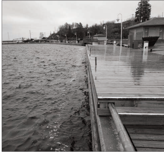
Last year's record high water levels caused the Northeast Town to place platforms atop their downtown docks. While this year's levels are still high, they are 35 centimetres below last year's levels at this time.
