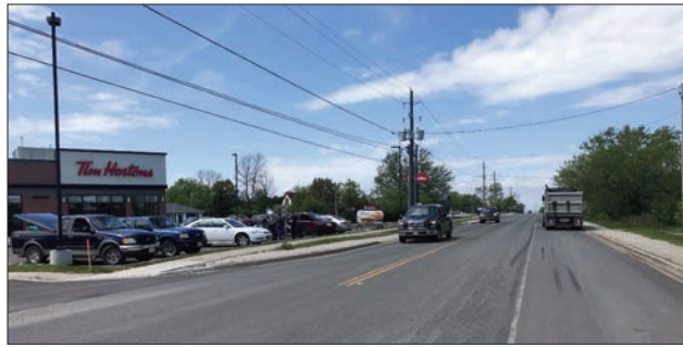
Parking in the far right-hand lane will soon be a thing of the past as this lane on Manitowaning Road is set to become another passageway for northbound traffic in the hopes it will alleviate summer bottleneck concerns.
