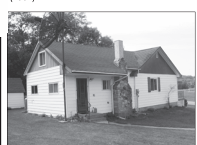
GORE BAY HOME on corner of Bay & Water Streets w/full view of water, parkland & marina. Bungalow 1356 sq. ft. w/spacious living room, dining area w/stone fireplace, kitchen, bath & large bedroom on main level plus loft bedroom w/bath. Extras include decking, sheds & appliances. $140,000 (1452)
