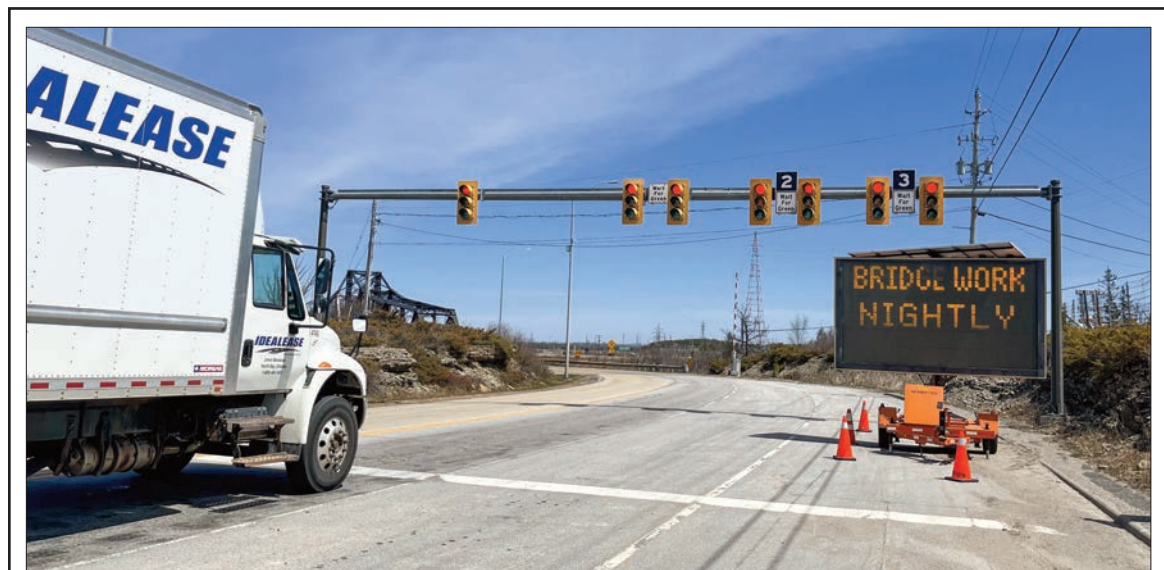
Evening work begins on swing bridge
