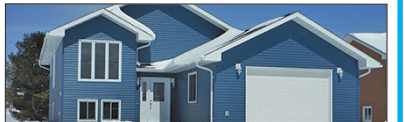
MINDEMOYA - New home construction by local reputable builder in a desirable location. 3 bedrooms and 1 full bath on the main level. Large open concept kitchen, dining, and living room. The lower level is unfinished with unlimited potential. Ceilings are over 8' and roughed-in plumbing for a bathroom. List price $226,900. MLS#1036505
