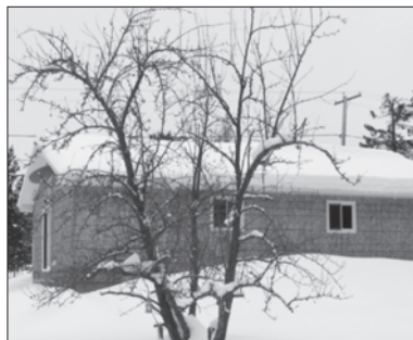
NEW COUNTRY HOME on east side of Silver Water being 1120 sq. ft. w/2 bedrooms, full bath, utility room & open area for kitchen dining living. Just built last fall, this work in progress, is finished to the vapour barrier w/200 amp service, electric & wood heat, full crawl space, drilled well & septic. Except for some furniture, everything stays including building materials, all construction tools, 5 appliances, generator, bunkie & shed. Take a look. $129,000 (1441)
