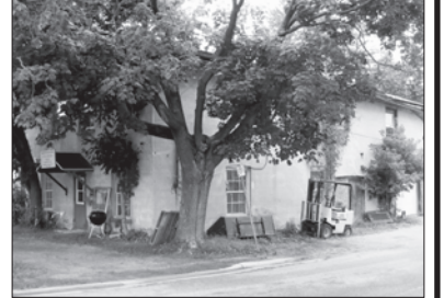
BLACKSMITH CENTRE on corner of Main & Meredith Streets w/4320 sq. ft. over 2 floors. Concrete building 36x60 ft. on fully serviced 39x127.6 ft. lot zoned core commercial. First floor garage plus business space & second level 4 & 1 bedroom apartments. $119,000 plus HST (1432)
