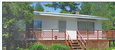
CENTRAL MANITOULIN HUNT CAMP - Hunt camp on 100 acres in Central Manitoulin. 900 sq.ft. camp with 3 bedrooms, wired for a generator, large deck, and with a fireplace insert. Trails, roads, and tree stands on site. Fronts on OFSC trail system. Most contents remain. Great price at $100,000. MLS#1032072
