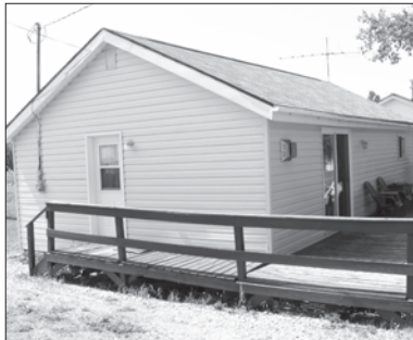
LAKE MANITOU COTTAGE on level lot w/60 ft. Rockville Road waterfrontage, sandy beach, good dock & sand bottom swimming. Bungalow 754 sq. ft. w/deck across water side has 2 bedrooms, 4 pc. bath, open kitchen dining living area w/propane stove fireplace. Recent upgrades of windows, doors, siding, shingles, fascia, soffits. Most contents including newer washer, refrigerator, stove. $154,000 (1431)
