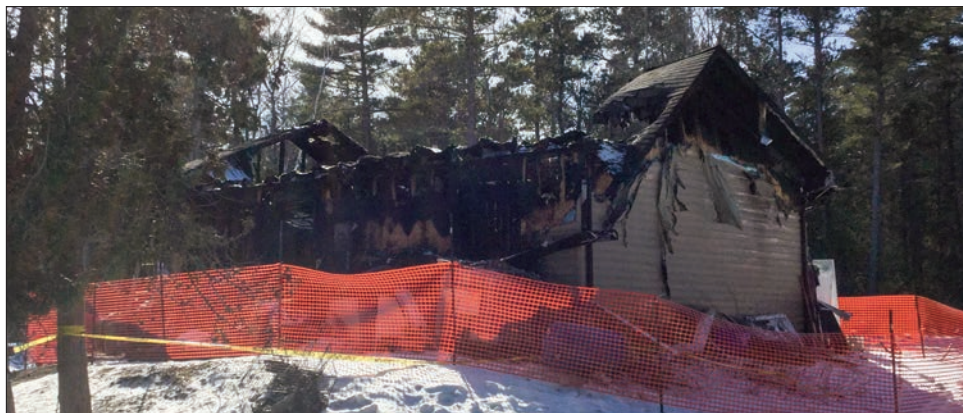
This is the former home of Whitefish River First Nation resident Evelyn Jacko. A GoFundMe page has been set up to help the fire victim.
