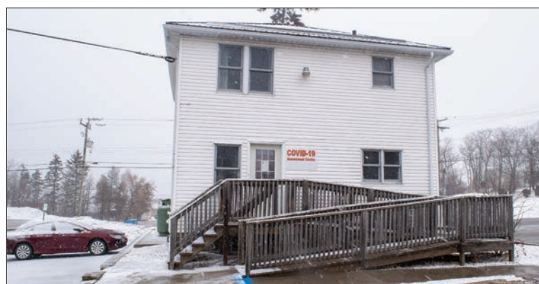
The Little Current COVID-19 assessment centre is located on the hospital grounds in the former withdrawal management services building.
