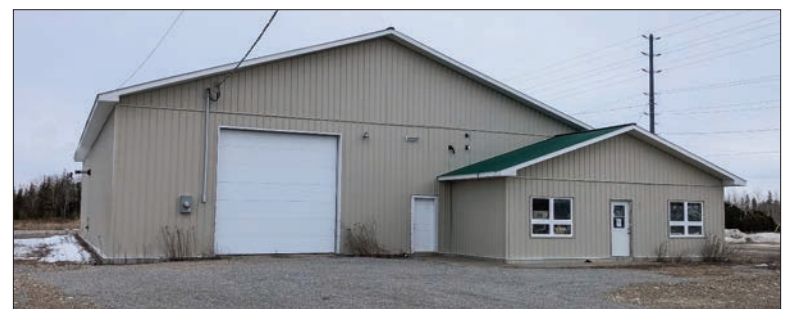
This building will soon be the new home of the Little Current fire hall. The new location is two to three times larger than the current hall.
