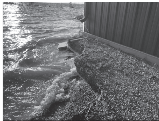
Record-high water levels compromised Zhiibaahaasing's existing water treatment plant's structure. A new permanent plant is needed.
