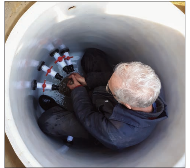
The scale of the forest sap reservoir is evident as Mr. Burt gets down inside to make the final connections on the pipelines before washing out the container to be ready for this season's bounty.
