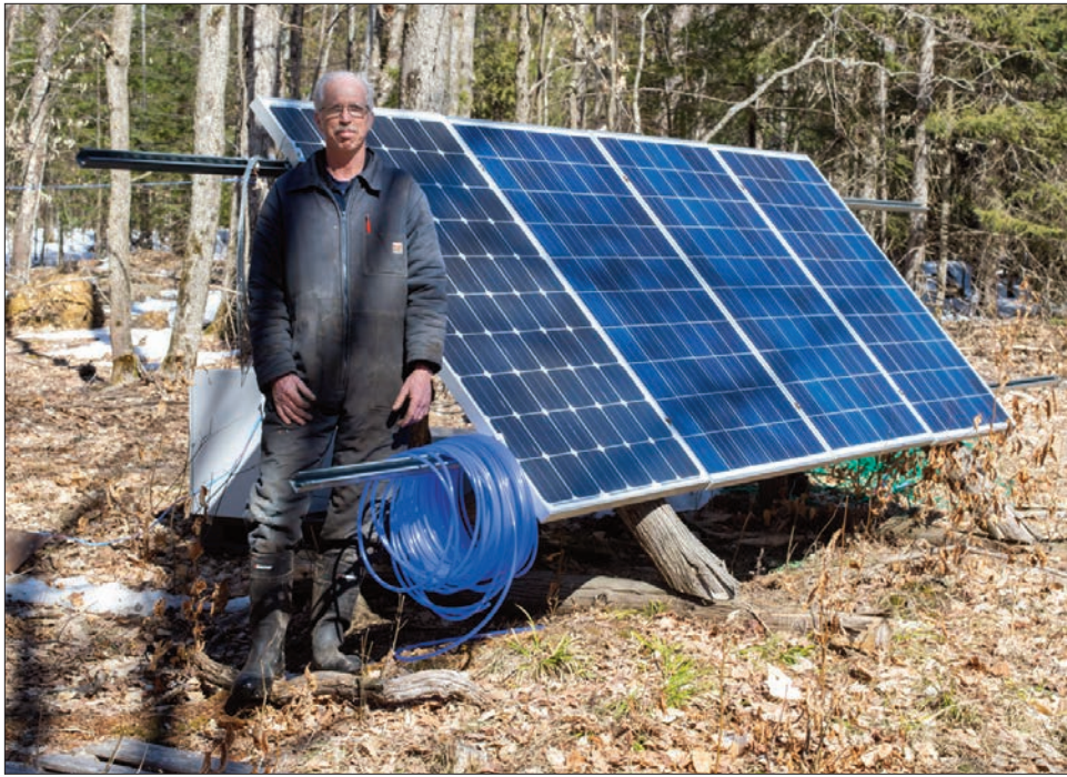
Ice Lake farmer Max Burt has created a fully off-grid system to automatically gather and send gallons of maple sap up to his sugar shack near the top of his property. The pump runs off this solar array.
