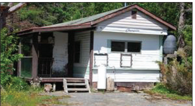
300 ACRES WITH HUNTING CAMP - near Hwy 542 in Campbell Township on Pine Tree Trail across from Union Road. Accessible by vehicle on unopened road allowance. The camp is well organized with wood heat, propane range, wood fired sauna with shower & sleeping quarters for as many as ten. The property is set up for deer hunting with many trails & tree stands. A Hydro Line runs right past the camp if the new owners are so inclined. This property could also be used for summer recreation such as ATVing or for those who just like to get away & camp. Reduced to $164,900. MLS#2060989
