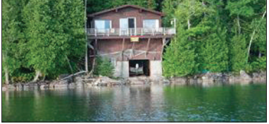
A VERY UNIQUE & CHARMING SUMMER HOME ON LAKE MANITOU - This property consists of a modern summer home with all the conveniences; a restored log building with a huge living/recreation room with a large stone fireplace, pool table & large covered verandah overlooking the lake; & a second log building which could be used as a bunkhouse. The main cottage has a boathouse underneath with a rail system into the water. The lot consists of 486 ft of frontage & 1.7 acres with an amazing view over Lake Manitou. This property comes completely turn-key including all appliances, furniture, dishes, cooking utensils & even a boat & motor. Reduced to $285,000. MLS#2061213
