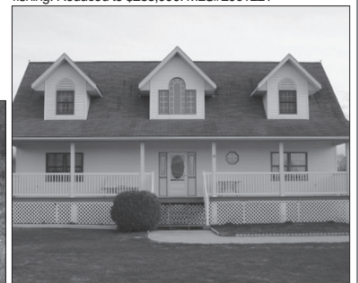
EXTREMELY HIGH QUALITY 3 BDRM HOME WITH NICE VIEW OVER LAKE MINDEMOYA!! - This beautiful home with its hardwood floors & vaulted ceilings comes with a magnificent kitchen with cherry stained maple cabinets, 3 baths including the en-suite in the huge 600 sq ft master bdrm located at the top of a spectacular oak stair case. The manicured lot comes adorned with a variety of mature trees which nicely outline the property, amazing concrete driveway & huge sidewalks leading to 2 large decks of which one is a covered verandah. Also on the lot is a 10 x 12 storage shed & a heated completely finished & insulated double size garage. Asking $370,000. MLS#1037157
