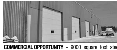
COMMERCIAL OPPORTUNITY - 9000 square foot steel frame and clad building currently used as auto/marine repair shop - 5 x 14' bay doors and 1 10' bay door. In floor radiant heat, fully insulated shop. Ideal for many uses including auto/marine/rv/rec vehicle, indoor heated storage facility and so on. 3 acres of useable land. Municipal water to property (not connected at present). Great location and easy access off Hwy 6. Great potential for your business! $299,000. MLS#1029385
