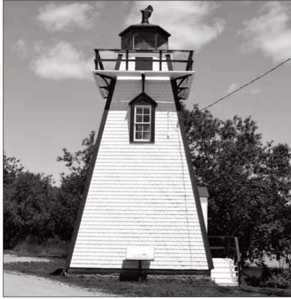
The Manitowaning lighthouse has had a facelift. The photo on the left shows the lighthouse before the work, while the photo on the right was taken after the work was undertaken by the Department of Fisheries and Oceans over the last three weeks. The work included the scraping off of the old paint, the repaint and trim touch up. The DFO also replaced the plexiglass found in the tower with glass.
