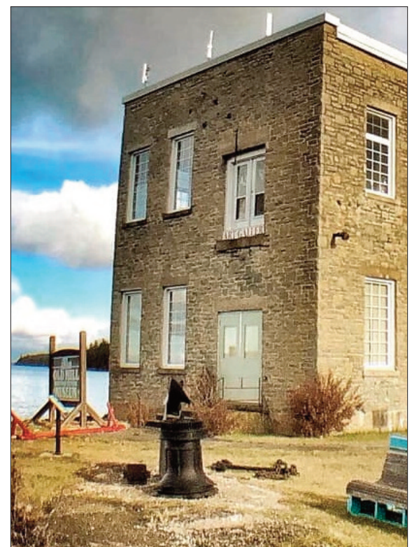
The Old Mill Heritage Centre sports a new side entrance that is separate from the municipal office.
