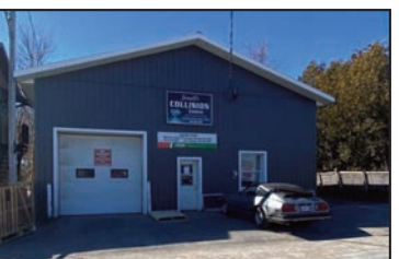
Mechanical Garage Building & Business MLS®#: 2092721, $499,000
