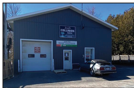
Mechanical Garage Building & Business MLS®#: 2092721, $499,000
