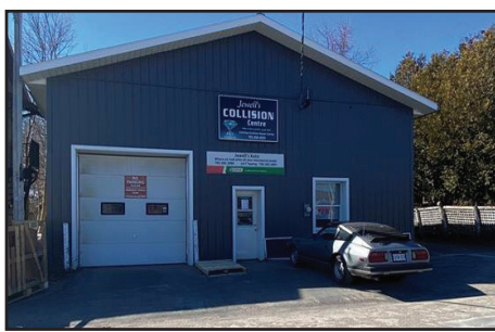
Mechanical Garage Building & Business MLS®#: 2092721, $499,000
