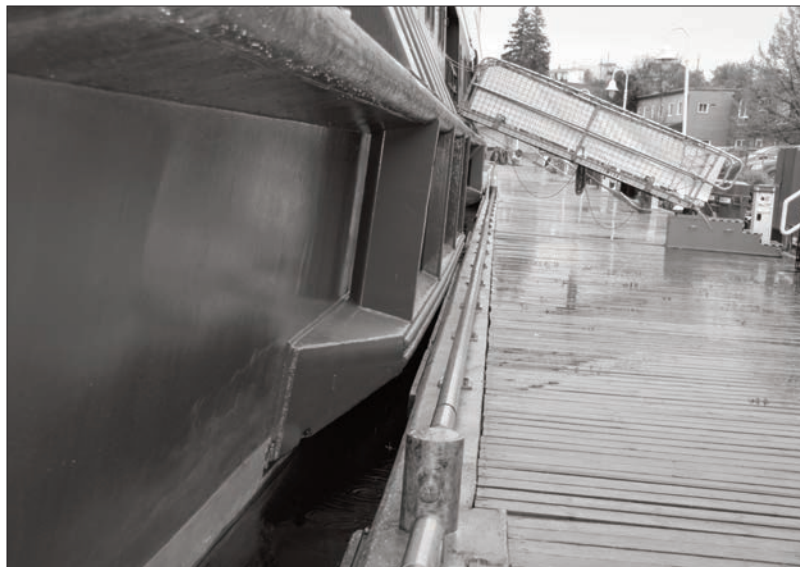
The fixed steel bumpers on the Victory I cruise ship caused damage to Little Current's docks last week due to high Lake Huron water levels.
