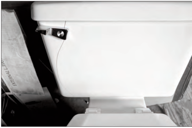
This toilet in the Auberge Inn in Providence Bay was cracked, reportedly after tremors rocked the area.
