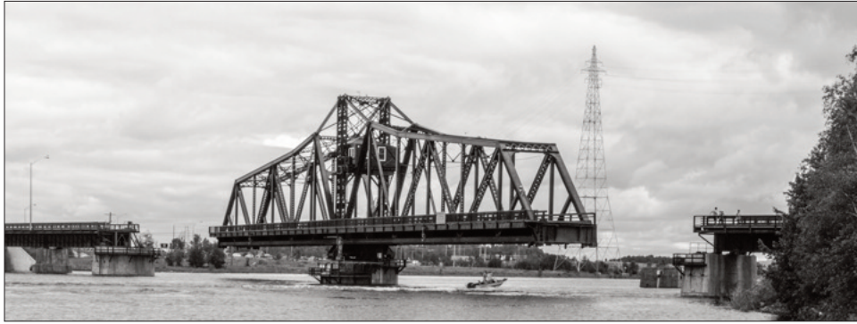
The fate of the famed Manitoulin Swing Bridge is under review.
