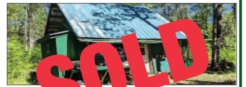
MAPLES POINT on a large lot, fronting on, year round, McQuarrie Road w/ access to the lot line. One room cabin plus screened room, privy, wood shelter & driveway, ready to camp in comfort. Access to the North Channel just down the street to Range A Sideroad. Great escape! $89,000 (1531) (MLS #2096973)
