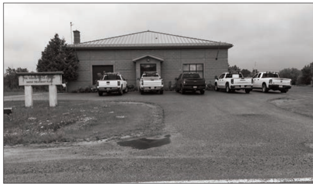
Extra technicians from Ontario Clean Water Agency were on the scene of the Little Current Water Treatment Plant Saturday.
