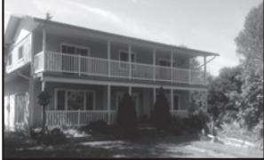
CENTRALLY LOCATED LITTLE CURRENT HOME
