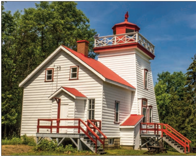
The Janet Head Lighthouse was built at Gore Bay's entrance in 1879 in the 'Georgian Bay' style; it accommodated a lighthouse keeper and family in living quarters attached to the light tower.
