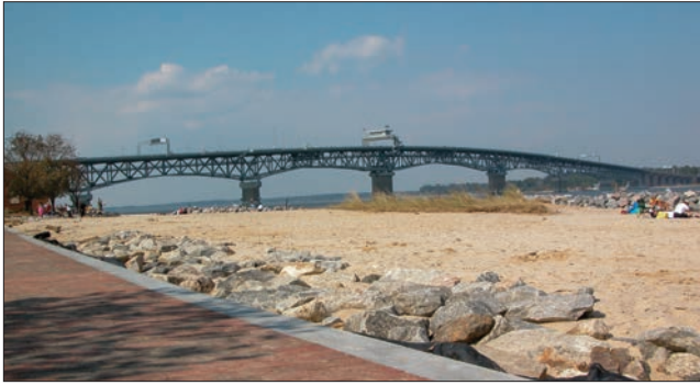
The George P. Coleman Memorial Bridge that spans the York River, joining the communities of Yorktown and Gloucester Point, Virginia is the largest swing bridge in the US and was replaced in only nine days.
