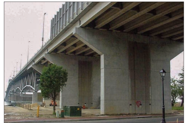
The Virginia bridge boasts massive abutments.
