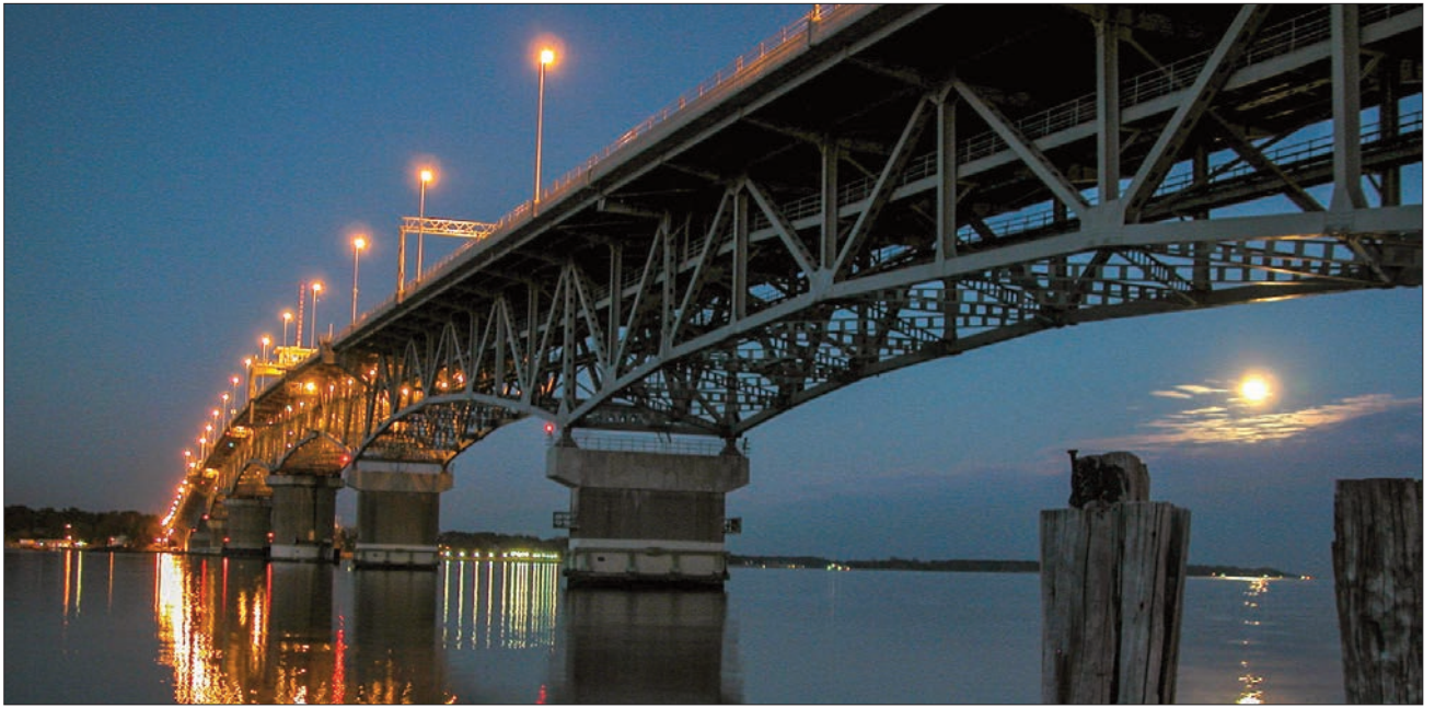
The George P. Coleman Memorial is America’s largest double-lane swing bridge at 3,750 feet long (and second largest in the world) and supports four lanes of traffic.
