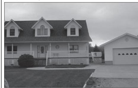
EXTREMELY HIGH QUALITY 3 BDRM HOME WITH NICE VIEW OVER LAKE MINDEMOYA!! - This beautiful home with its hardwood floors & vaulted ceilings comes with a magnificent kitchen with cherry stained maple cabinets, 3 baths including the en-suite in the huge 600 sq ft master bdrm found at the top of a spectacular oak stair case. The manicured lot comes adorned with a variety of mature trees which nicely outline the property, amazing concrete driveway & huge sidewalks leading to 2 large decks of which one is a covered verandah. Also on the lot is a 10 x 12 storage shed & a heated completely finished & insulated double size garage. Asking $370,000. MLS#2074309
