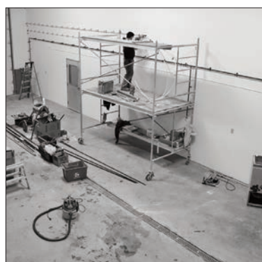
The third garage and attached office, lunchroom and storage area can be heated separately from the other side of the building, which houses the additional two-bay garage.
