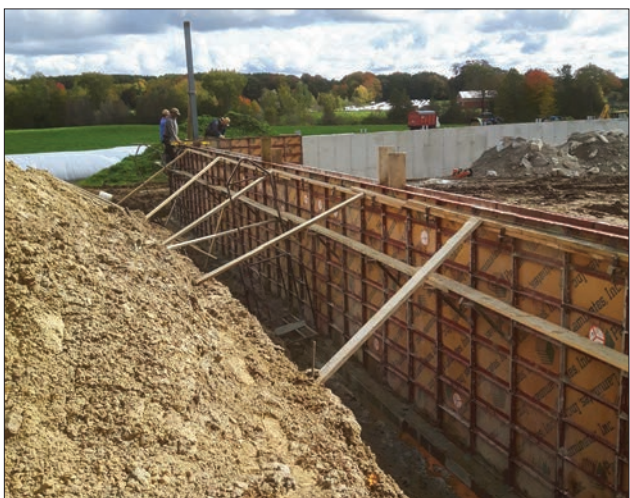
Footings for the new barn were poured on September 29.
