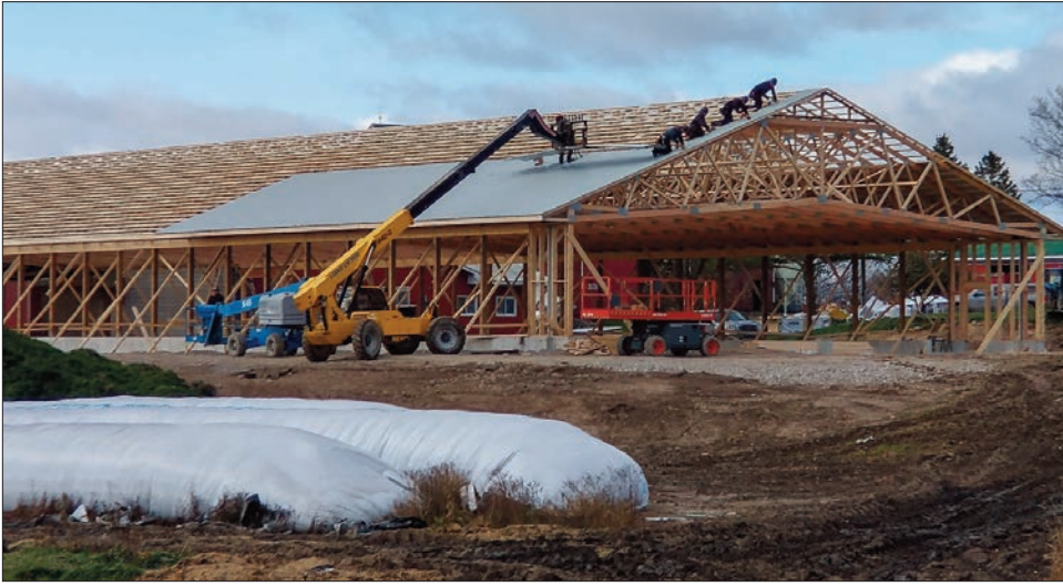
Metal roofing is placed on the state-of-the-art Tehkummah barn on October 30.
